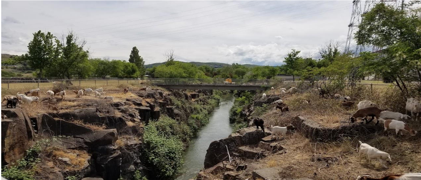
Goat successfully removing vegetation from upper channel. Limitations to waterline access.
